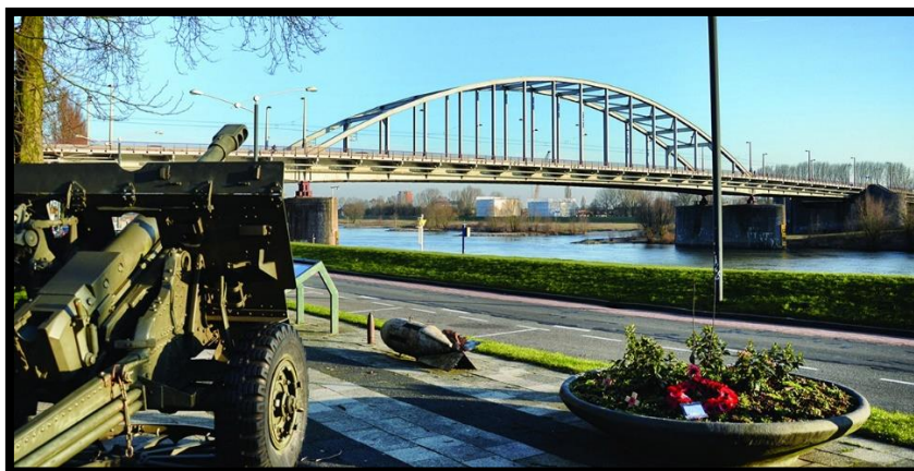
Sl. 19. Arnhem Bridge
