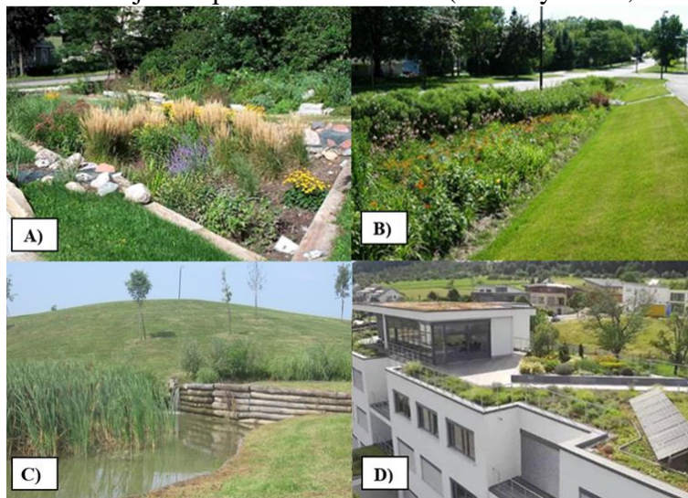
Slika 3-1 : Primjeri prirodnih rješenja A) kišnog vrta ( https://www.esf.edu/ere/endreney/GICalculator/RainGardenIntro.html ), B) jame za odvodnju oborinskih voda ( https://stringfixer.com/tags/bioswales ), C) retencijskog bazena ( https://unalab.eu/system/files/2020-02/retention-basins-and-draining-areas-genovas-water-webinar-contribution2020-02-17.pdf ) D) zelenih krovova ( https://www.geoplastglobal.com/en/blog/interesting-green-roof-research-articles/ )
