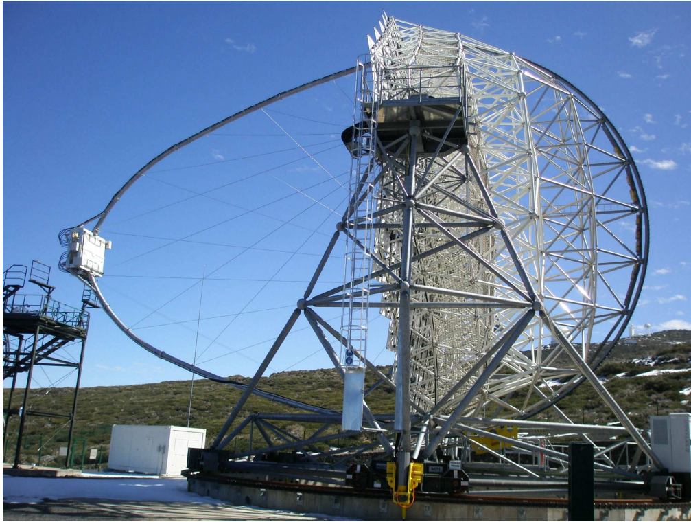
Figure 2.2 Side view of the MAGIC-I telescope. The construction of carbon fibre reinforced plastic tubes is white, and the lower part constructed of steel bars is grey. On the left, camera is supported on aluminium mast. A web of steel cables is also visible.
