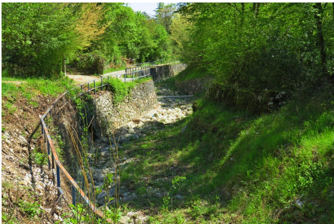
Sl. 61 Reguliran donji tok bujice u Medveji
