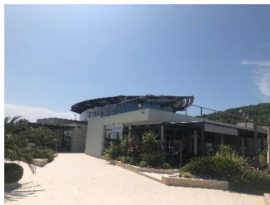
Sl. 6. Zgrada marine Olive Island
