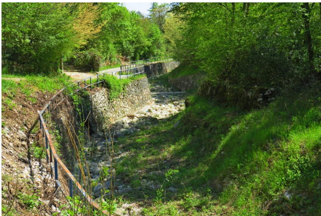
Sl. 61 Reguliran donji tok bujice u Medveji
