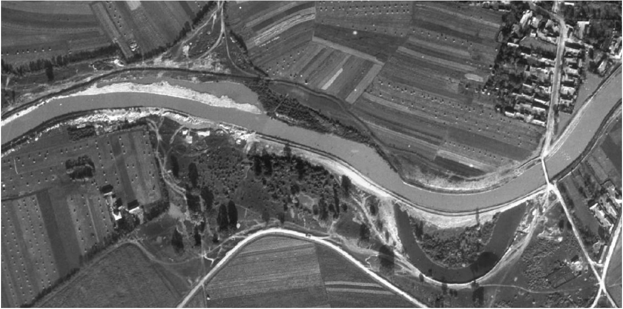
Figure. 3.1.12. An example of Bednja River training underway at Veliki Bukovec as seen on satellite imagery from 1968 (scale 1:2000). Image shows river width restriction works and meander cutting off (source: https://ispu.mgipu.hr/ accessed 21.03.2019).
