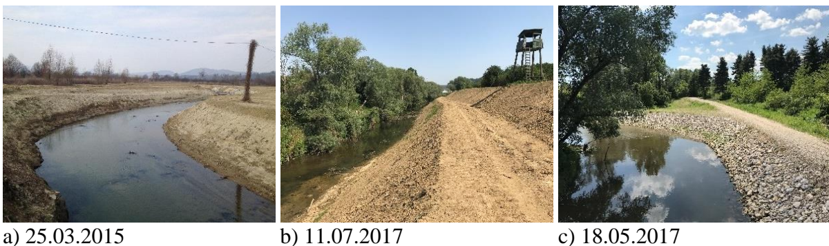
Figure 3.1.13. Regular management practices on the Bednja River: a) example where both banks are resectioned, Jerovec; b) example of single bank management, Novi Marof; c) bank reinforcement with “rip-rap”, Bednja downstream from Ludbreg.
