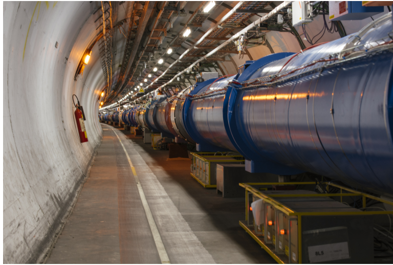
Figure 2.2: LHC tunnel situated underground which contains the LHC beam pipes
