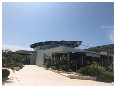
Sl. 6. Zgrada marine Olive Island
